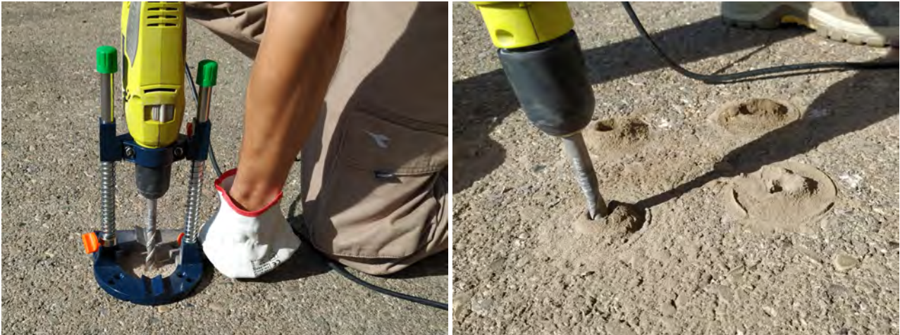
Figure : Drill the holes (step 1)
