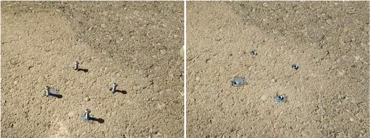
Figure : Final anchor installation (step 7)
