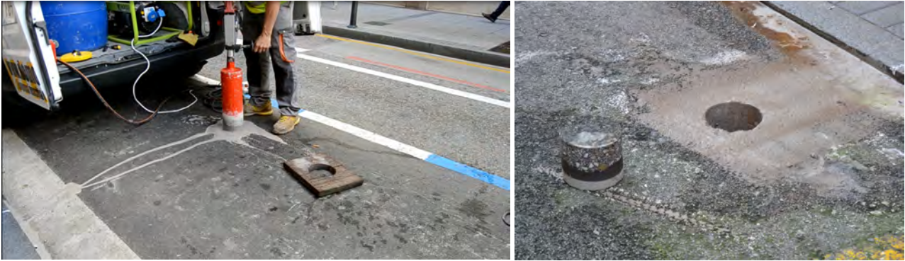
Figure : Making a hole in the pavement
