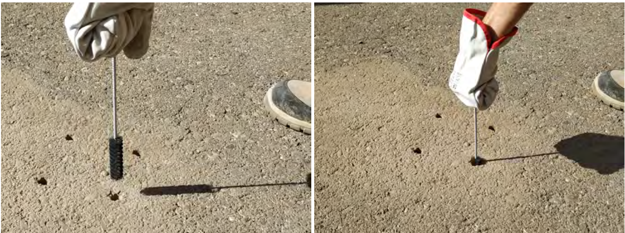
Figure : Brush the hole (step 3)
