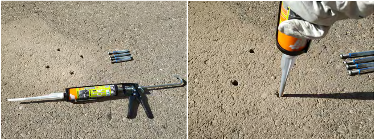
Figure : Inject chemical fixing adhesive (step 5)
