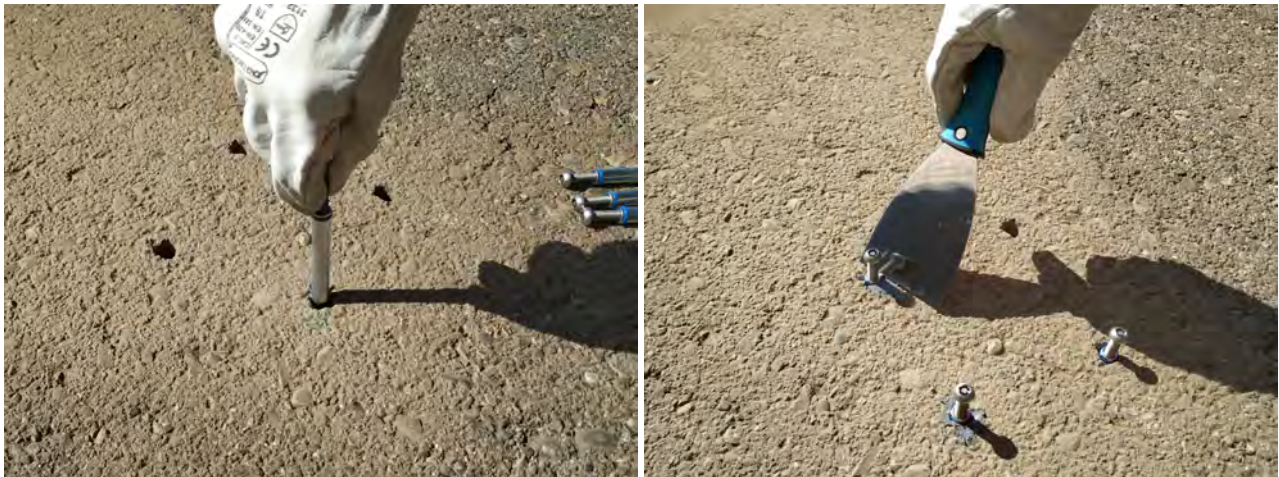
Figure : Insert the anchors (step 6)
